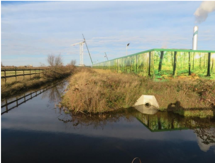
Photograph 2.1: An existing outfall from the compound into a ditch on the western and southern side of Borax North.
